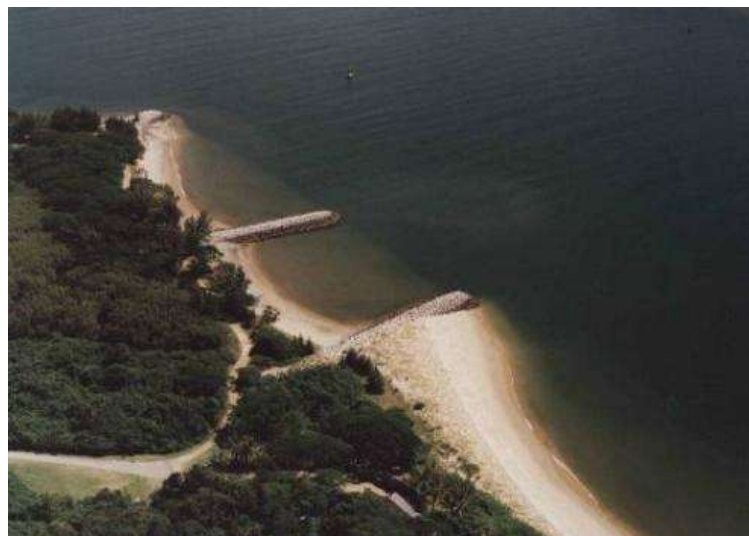
Figure 7.12: Groynes protecting Richards Bay entrance channel shoreline, South Africa (Photograph S Pillay)
