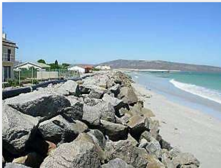
Figure 7.6: Example of a rock revetment protecting houses (South Africa)
