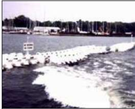
Figure 7.14: Patented floating breakwater ( www.whisprwave.com )
