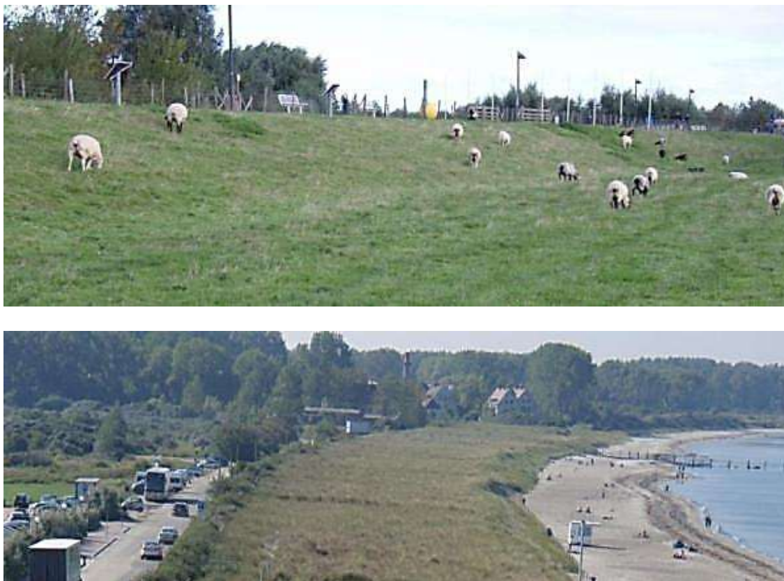
Figure 7.7: Examples of vegetated dikes (Germany)
