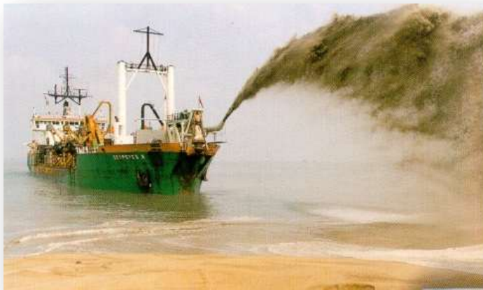
Figure 7.2: Beach nourishment by means of direct “rainbowing” of sand from the dredger to shore (only practical in certain areas).
