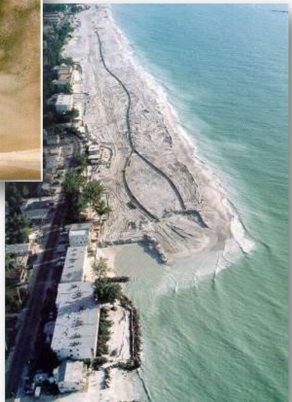
Figure 7.3: Beach nourishment by means of pumping sand onto the beach through a pipe system
