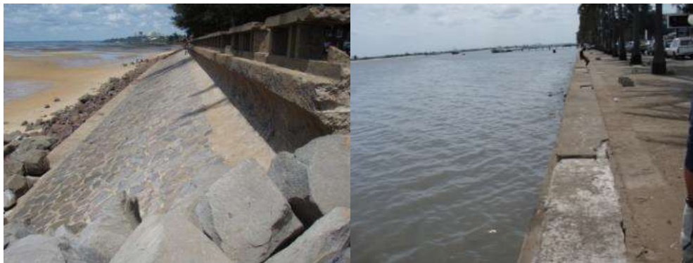
Figure 7.5: Examples of a revetment (left) and a seawall (right) in Mozambique
