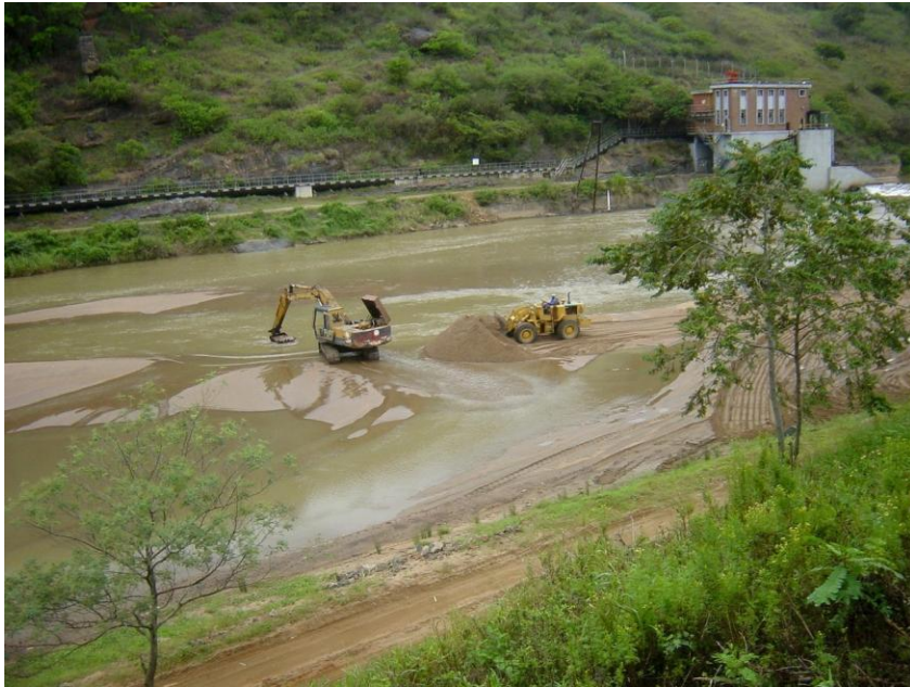
Reduction in sand supply due to sand mining
